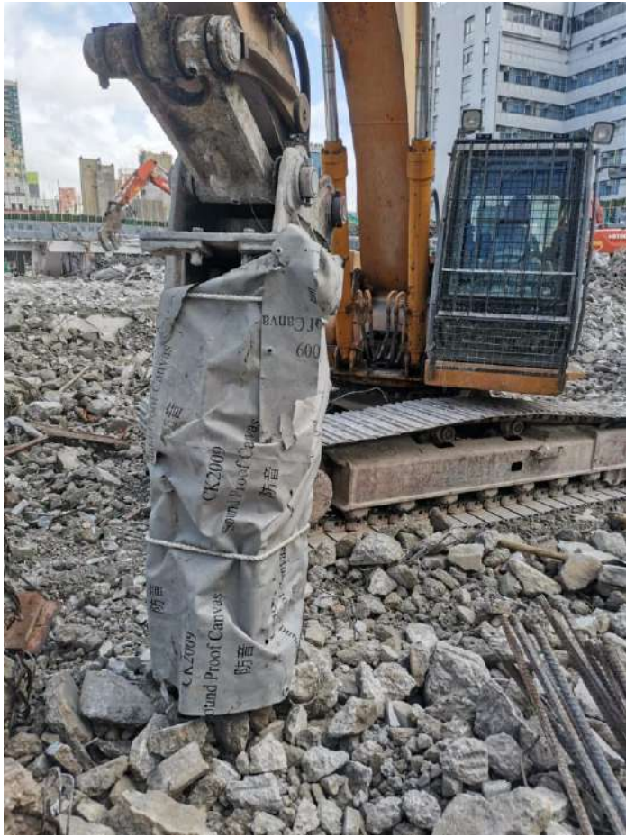
Figure A2: Breaker's tip wrapped with acoustic mat
